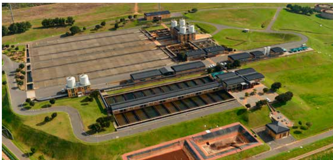
Faure Wastewater Treatment Plant is one of 27 such facilities serving Cape Town.
