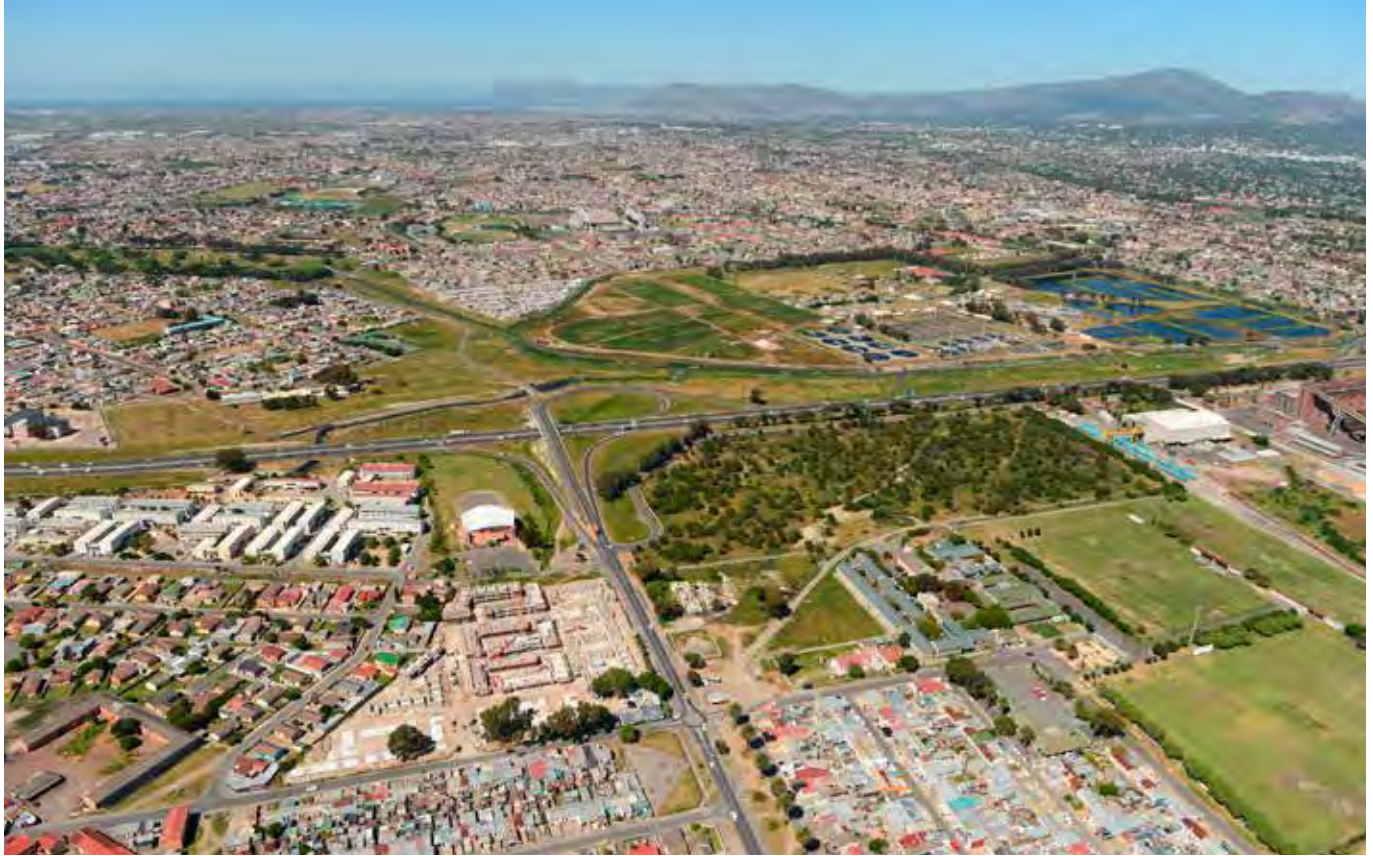
The Integrated Human Settlements Five-Year Strategic Plan defines the current housing reality in Cape Town.
