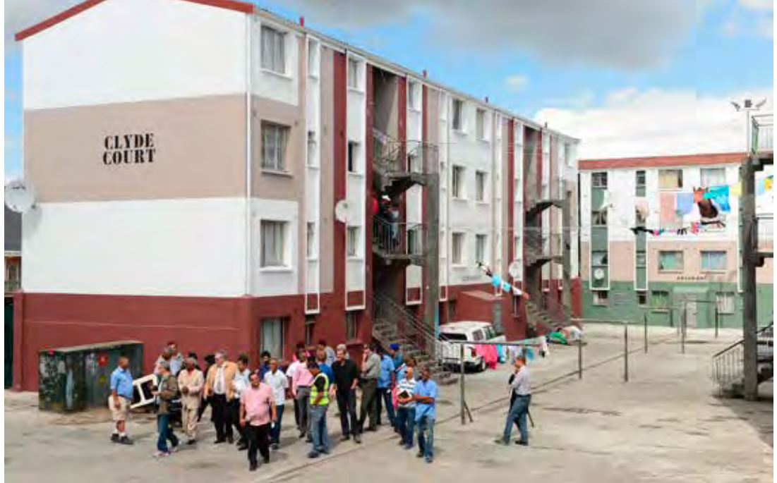
Upgrades to seven of the 11 identified rental stock have been completed.
