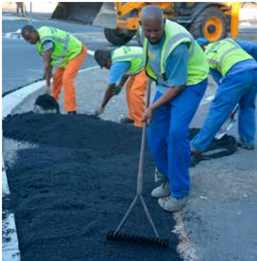
The City invested R2,9 billion in repairs and maintenance.
