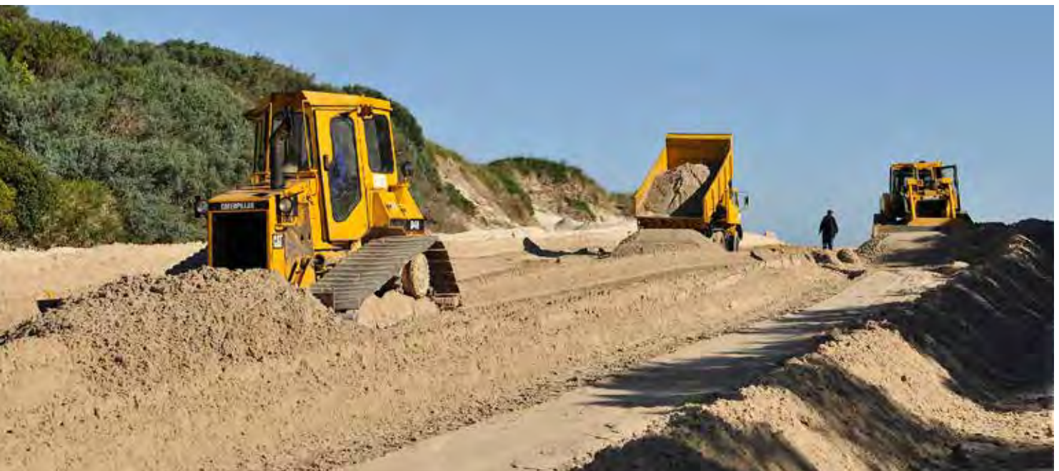
The Hout Bay dune management plan involves reshaping, planting and stabilisation of the dune system affected by urban development.
