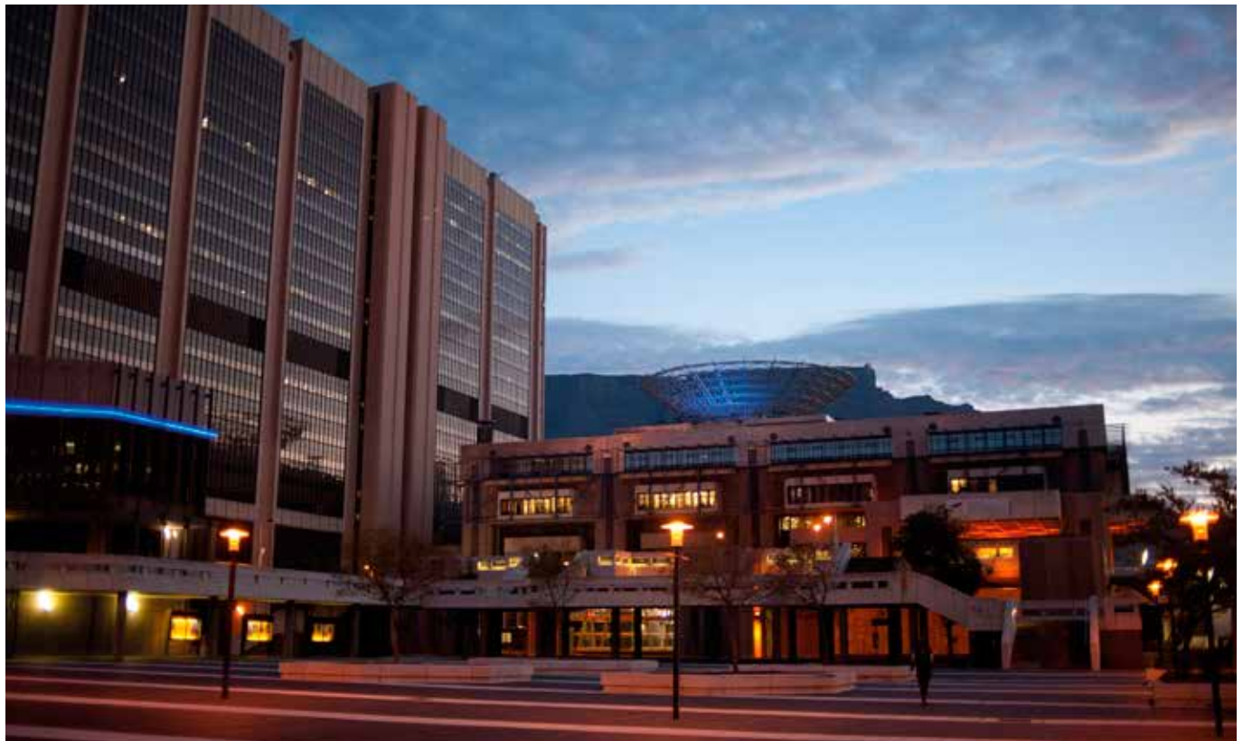
Cape Town Civic Centre, home to the political and administrative leadership of the City of Cape Town.
